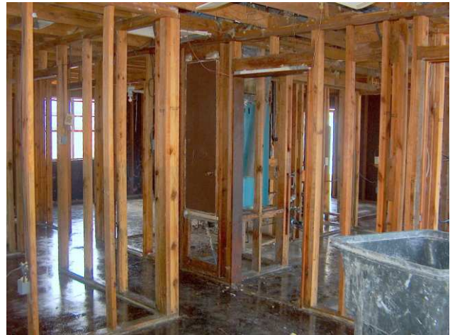
A gutted home ready to be re-built.
